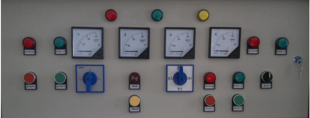
图 6-1 电控柜面板控制图 Picture 6-1 Controlling diagram of electric cabinet panel
